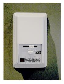
This space sensor is specially designed for Prolon VC500 and VC1000 controllers and can be mounted directly on a wall or to a box wall. For the most accurate results unit should be mounted on an inside wall, away from any air supply, exhausts and other source of heat or cold.
