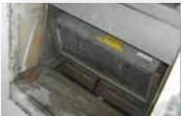
**4. Petri-dish Effect:** Warm, standing water in the drain pan can work like a giant Petri dish, cultivating bacteria and other potentially dangerous microorganisms; the equipment's fan then blows these microbes back into the building, degrading air quality and causing potential health problems.
